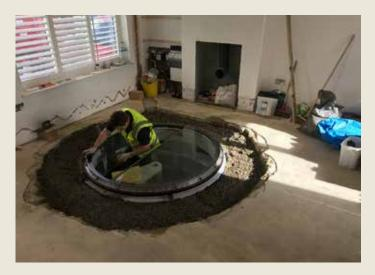
The cellar construction is then completed using Spiral Cellars' uniquely designed modular system of interlocking concrete bins and steps.
