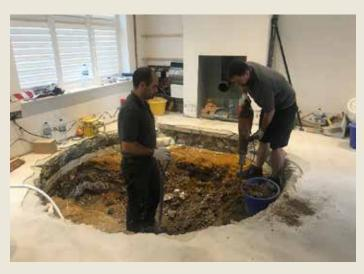
There is minimum disruption when installing a Spiral Cellar. The team excavates a hole in the room, two to three metres deep. They do so by hand which keeps noisy machinery off site – and the neighbours happy.
