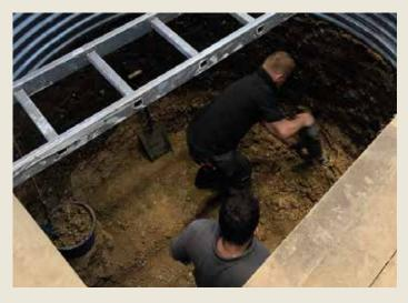
The hole is fitted with steel shuttering rings to give the cellar structure.
