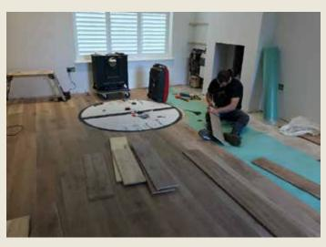
Additional items such as stair treads and LED packages are fitted to enhance the design and make the cellar a stunning feature in the room. The door is then carefully fitted and protected while the floor in the room is carefully re-laid and finished around the Spiral Cellar. Here the client has chosen a hinged round glass door.
