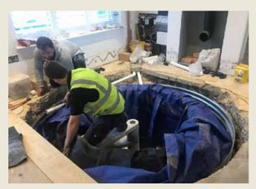
In turn, the ring is then lined with a robust waterproof liner.
