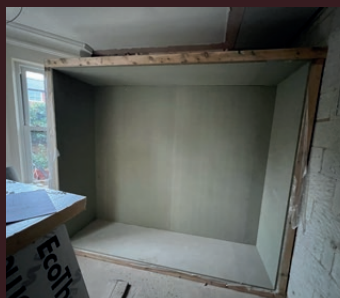
Structural frame erected
