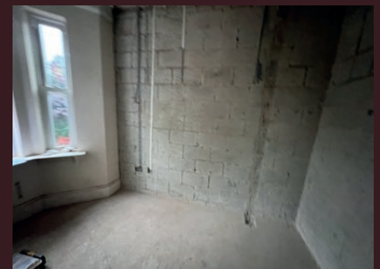
Wall stripped back ready for boxing and vapour control
